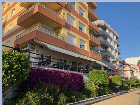
“Apartment building” by Yuriko Ikeda is licensed under CC BY 4.0
